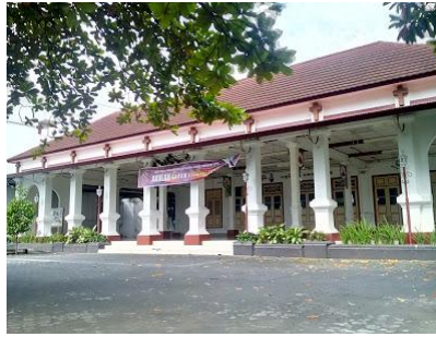
Figure 14 Paroki Orphanage Saint Yoseph Church Bintaran Designed with a Very Large and Relatively Large Front Porch its Elongated Building Forms to Accommodate Large-Scale Activities
