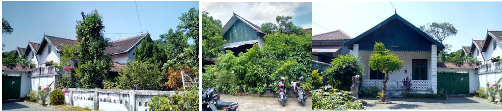
Figure 8 Appearance of Twin House Buildings that Characterized Indis as One of the Specific Architectural Works in The Bintaran Area
