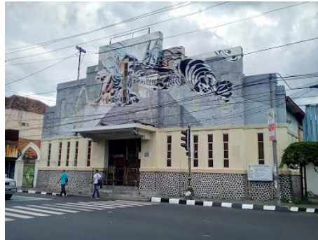
Figure 11 Former Permata Cinema, Currently is Not Functioned anymore, and the Condition is Getting Damaged in Line with the Age of the Build
