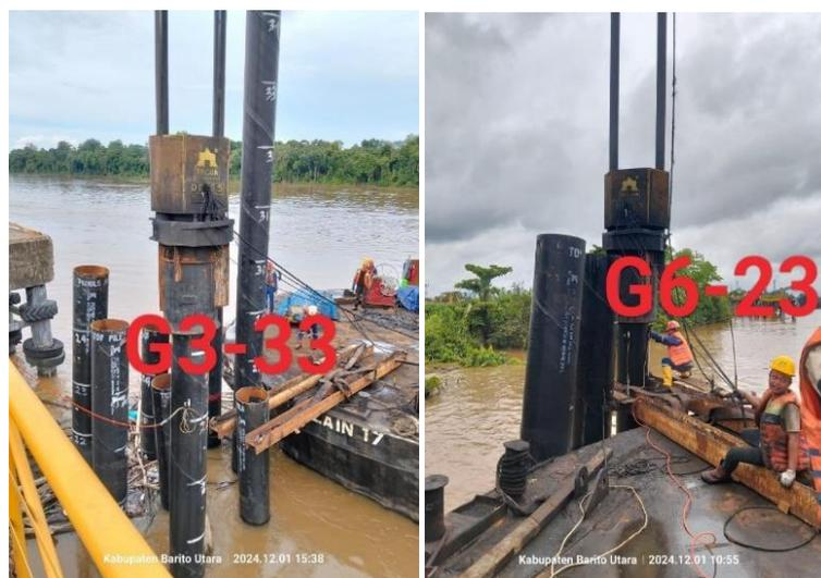
**Gambar 2.** Pengujian PDA Test SPP dia. 610 mm
