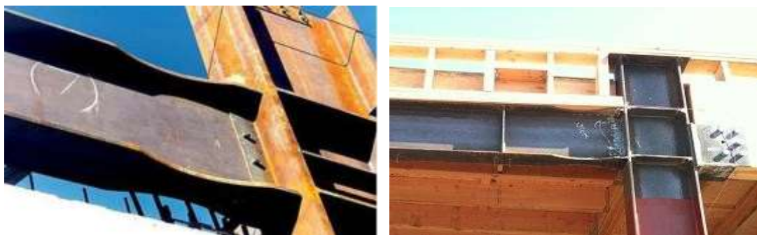
Figure 2. Application of Reduced Beam Section (RBS) Connection
